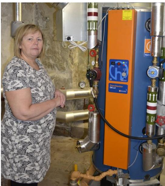
Since 2010/11, the project to upgrade Plas Maesincla has involved installing new heating controls, insulating heating pipes, upgrading the lighting system and installing new boilers. In addition, the home now generates its own electricity as a result of PV solar panels being fitted on the roof in 2014. All of this will enable the home to save £143,100 in energy costs and save 670 tonnes of CO<sub>2</sub>.
